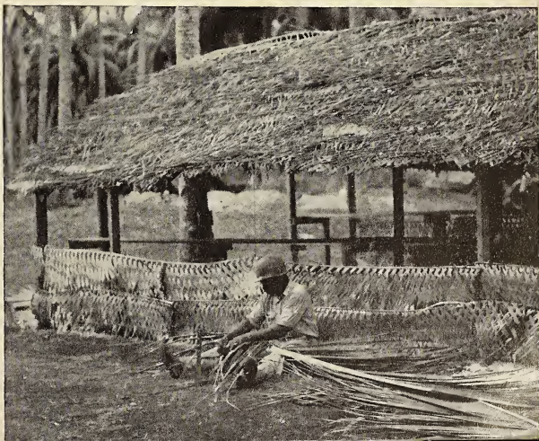
A butcher knife snatched from the mess hall helps this colored soldier expertly weave the walls of a new building from palm fronds.
